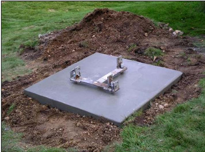
The freshly poured concrete base with the US Tower mounting hardware.
